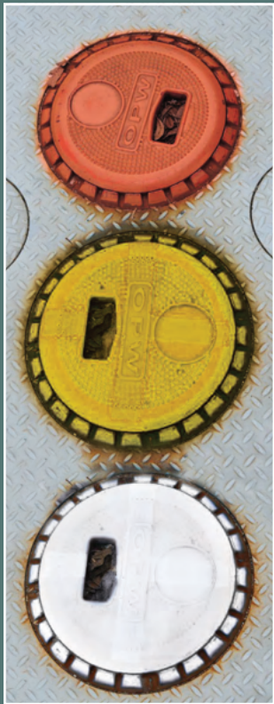
Spill bucket lids color-coded according to API 1637. From top to bottom: Premium E10 gasoline (red), Ultra Low Sulfur Diesel \leq 5\% biodiesel (yellow), Regular E10 gasoline (white)
